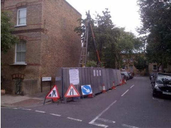
The gantry marks the surface expression of where the new tunnel, and the existing loop tunnel meet. A 6.5m high box will be excavated underground around the existing tunnel by hand, to facilitate the junction of the two tunnels. New Austrian Tunnelling Method, (NATM) dig a tunnel, spray with stabilising concrete then place new structural panels at a later time; is being used. This is the method that failed at Heathrow Airport
